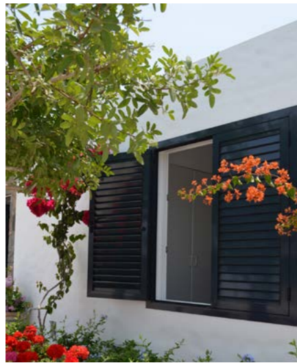
Closure with casement shutter and fixed slats.
