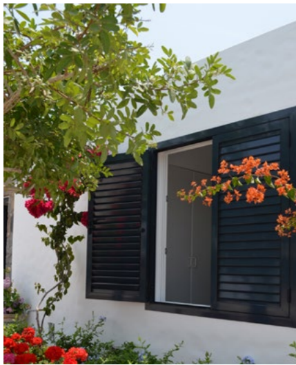
Closure with casement shutter and fixed slats.
