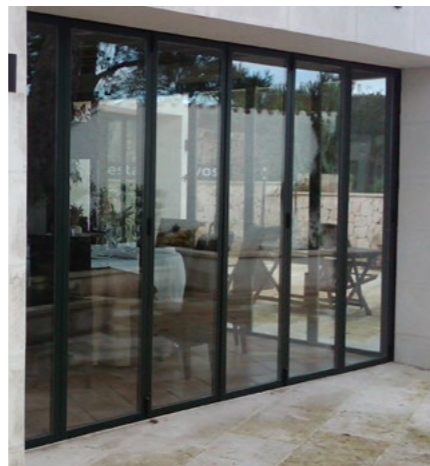
Shutter folding closure with 5 glass panels.
