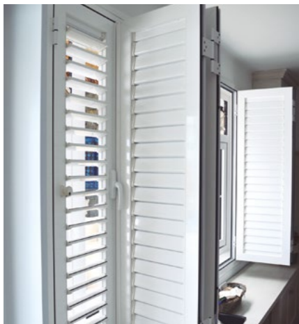
Shutter folding closure with movable slats.
